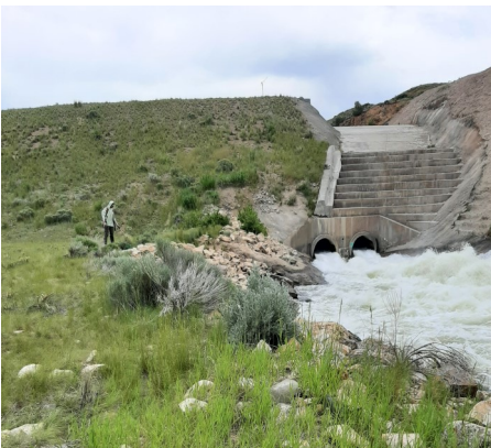
Mac spraying at Lima Dam- Shannon Wilkey
